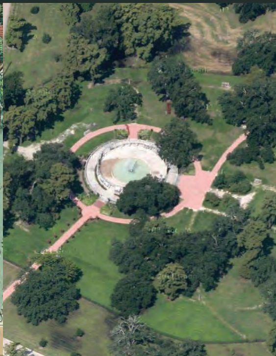
Popp Fountain Renovations (In Progress)
